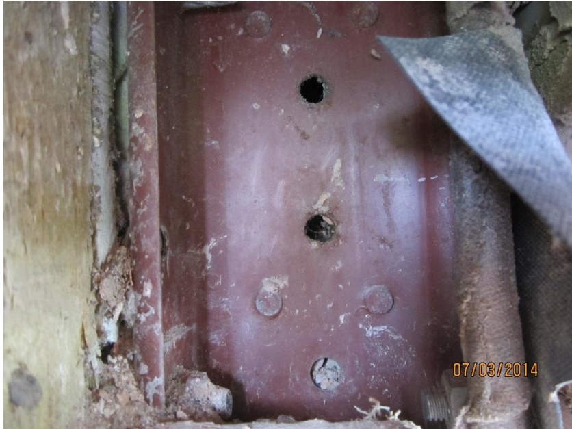
Column in Cavity
