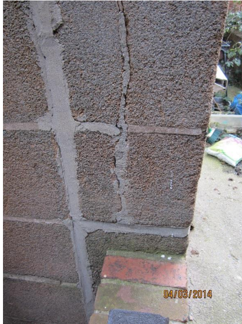
Cracked Panels
