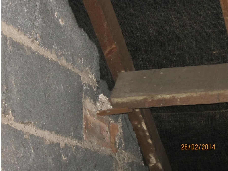
Poor Bearing for Purlin
