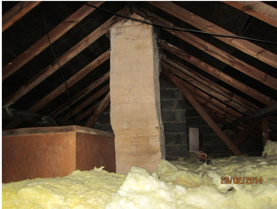
Poor Bearing for Purlin
