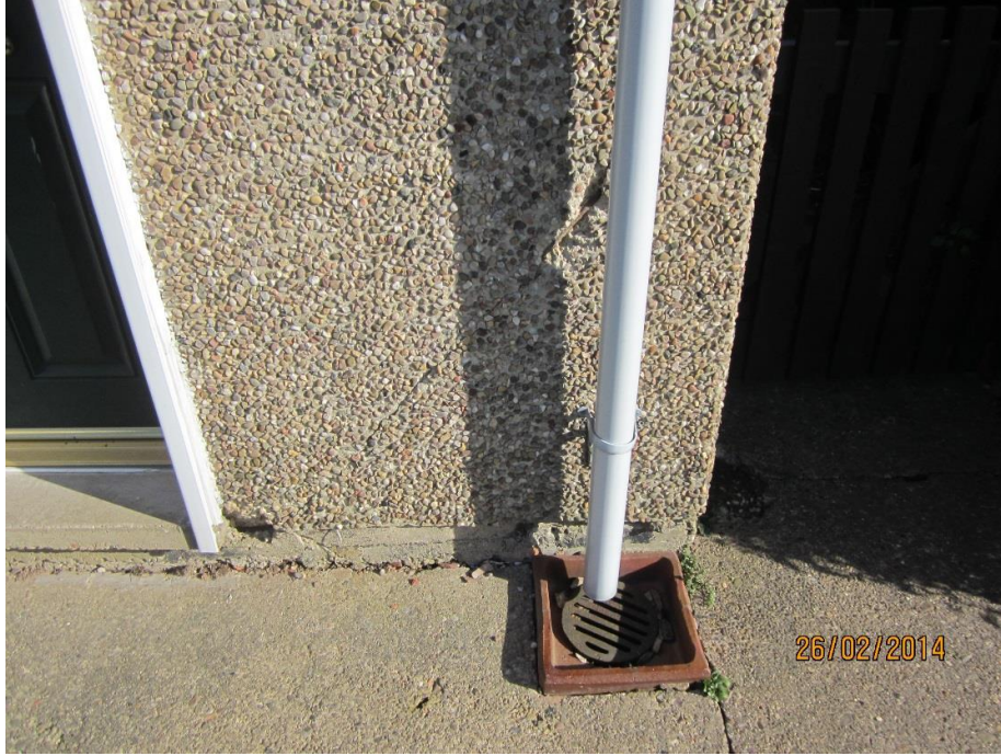
Cracked Panel
