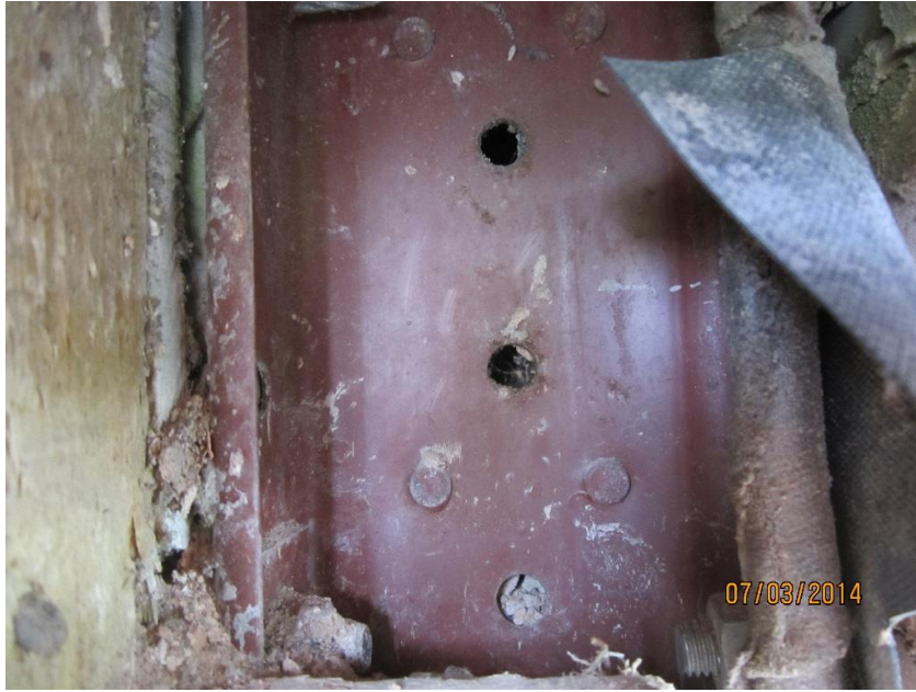
Column in Cavity
